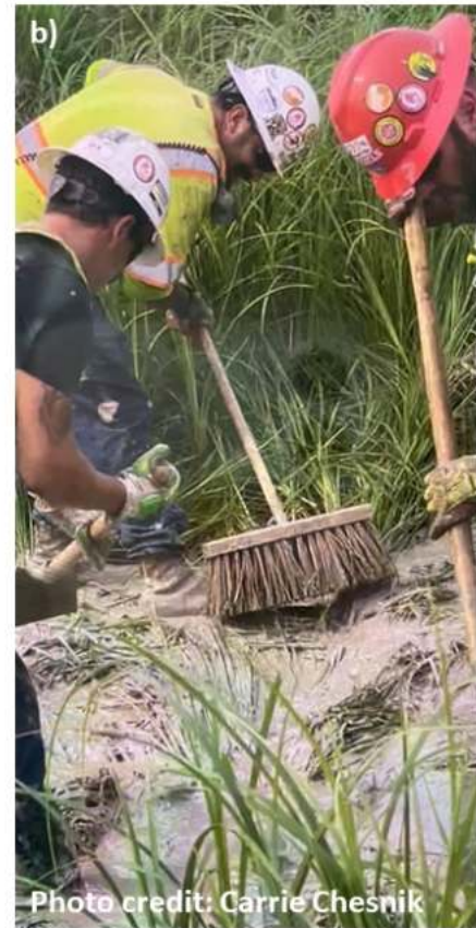
Figure 2. a) Top photo shows location of first known frac out at Mississippi River Crossing #1, observed by water protectors in a wetland on July 20, 2021. b) Right photo shows Enbridge workers attempting to clean up drilling fluid spill in the same wetland.
